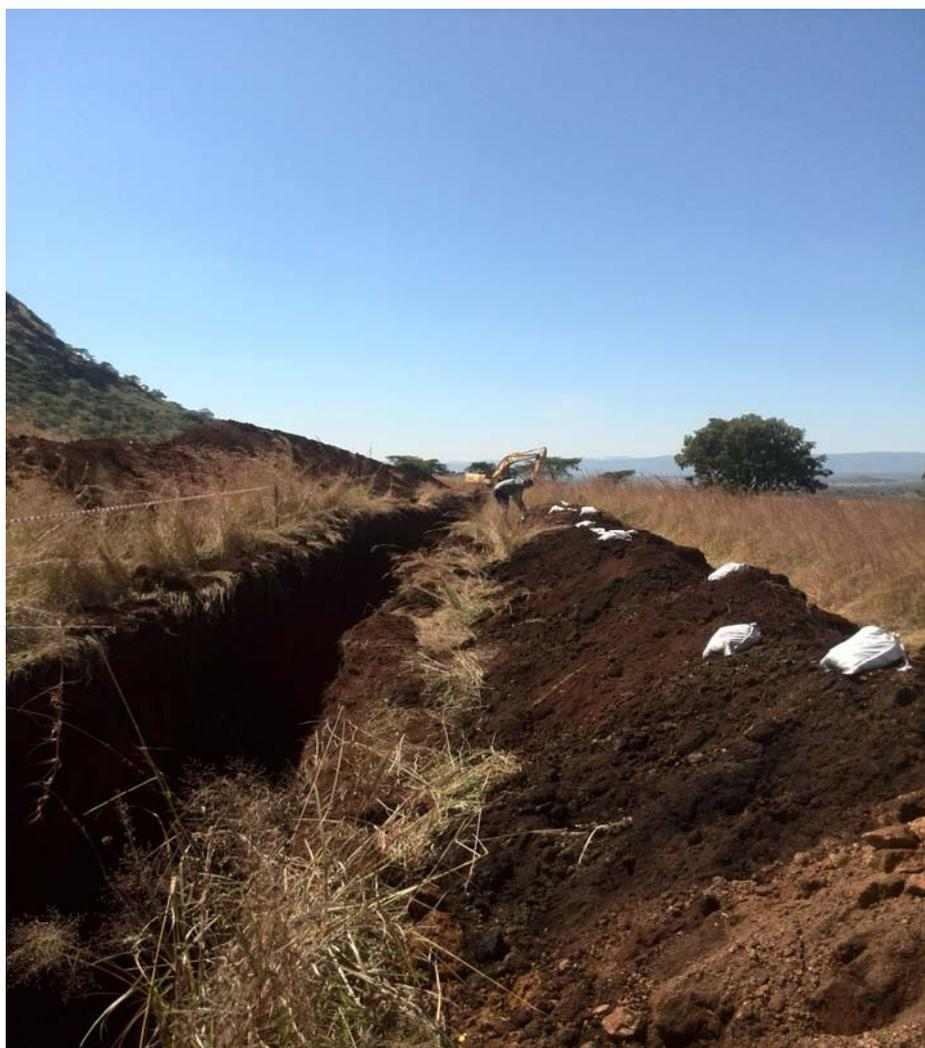
Fig 2: Trench sampling at Longonjo Rare Earth Prospect
